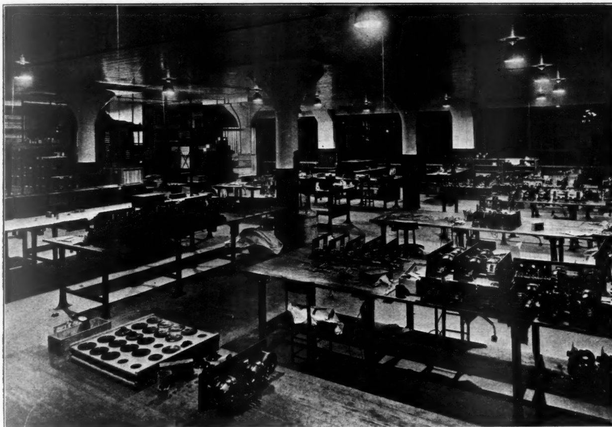
Modern illumination of a modern factory. A floor in the plant of A. H. Grebe & Co., manufacturers of radio sets at Richmond Hill, Long Island, N. Y. The bowls are silvered and reflect the light over measured overlapping areas.
